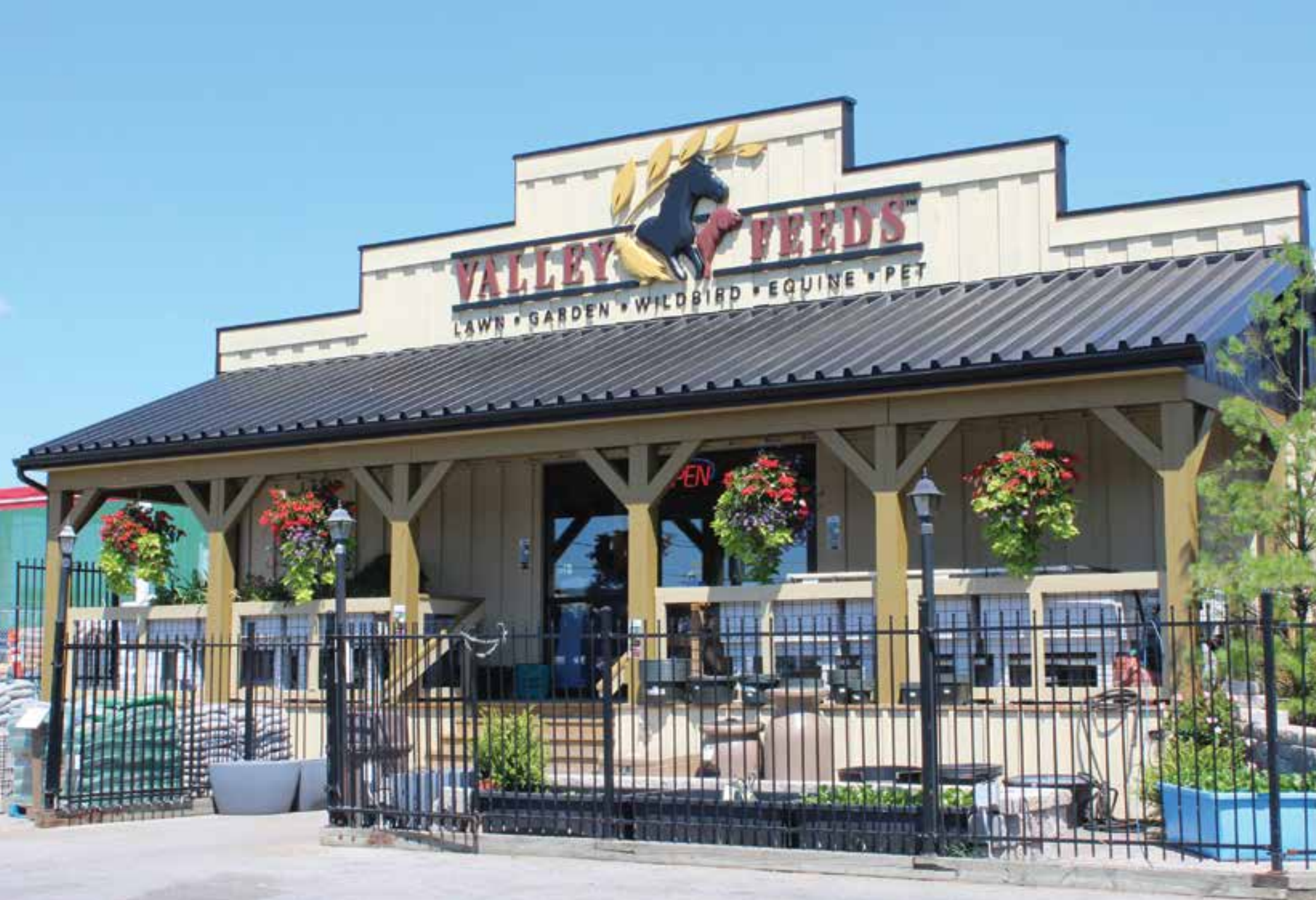
The new Valley Feeds store in Cambridge, Ontario, after renovations.
