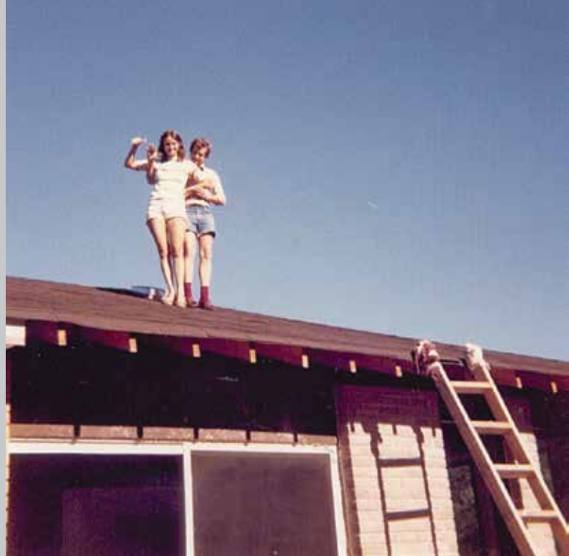
Ingrid and Wolfgang on the roof of their house while putting on an addition.
