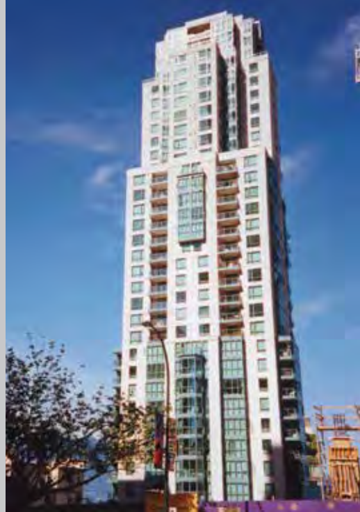
One of the high rises in Vancouver where Napoleon gas fireplaces were installed.
