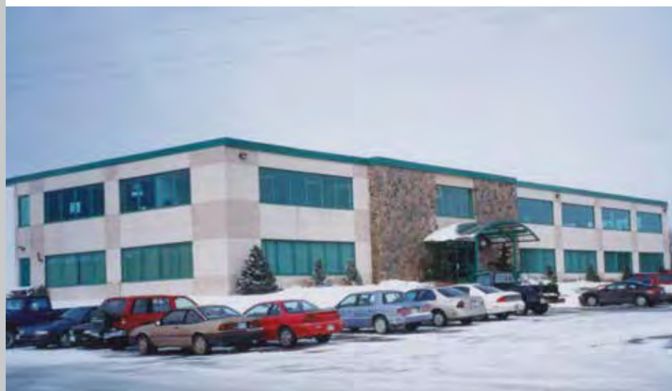
The NAC building after renovations.
