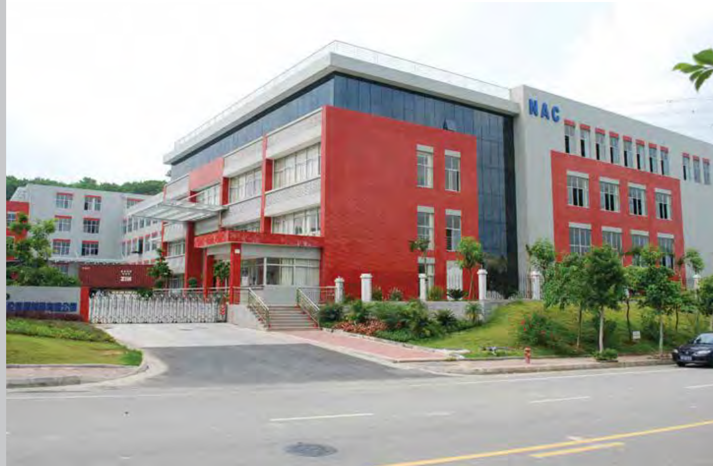
The Napoleon plant in China after completion.
