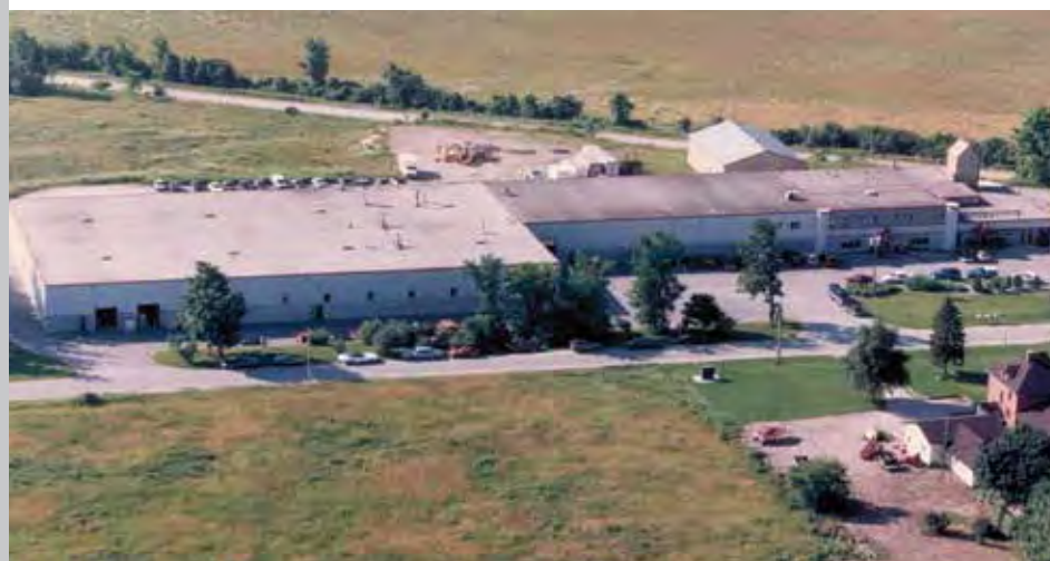
Second expansion to add production and warehouse space to the plant.
