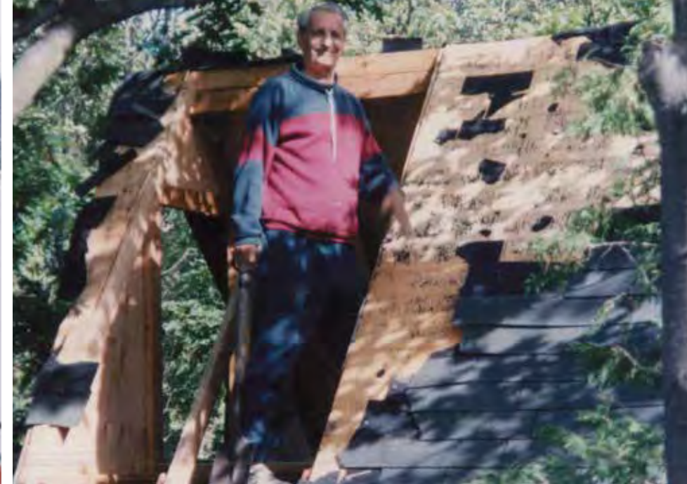
Ingrid's father finishing the roof of the family cabin on Rose Island.
