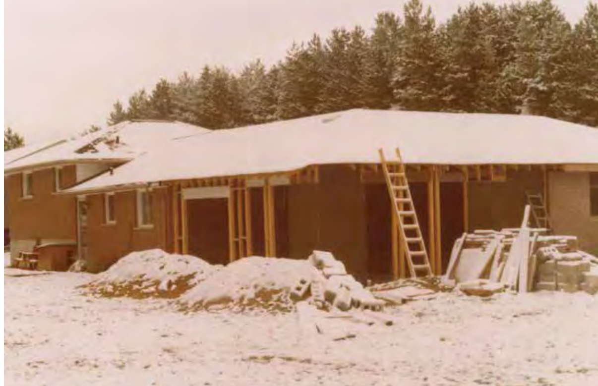
Ingrid and Wolfgang putting an addition onto their house in Utopia.
