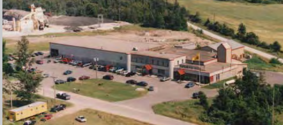
Adding production space during a plant expansion at 9 Napoleon Rd.
