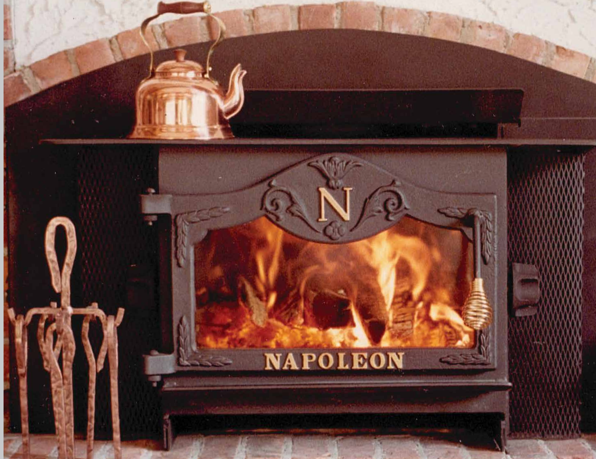
Napoleon insert installed in Ingrid and Wolfgang's home in Utopia.
