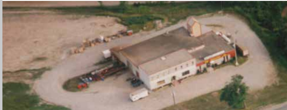
The plant on 9 Napoleon Road circa 1986 after adding a test tower, offices and a wholesale showroom at the front and a warehouse in the back.
