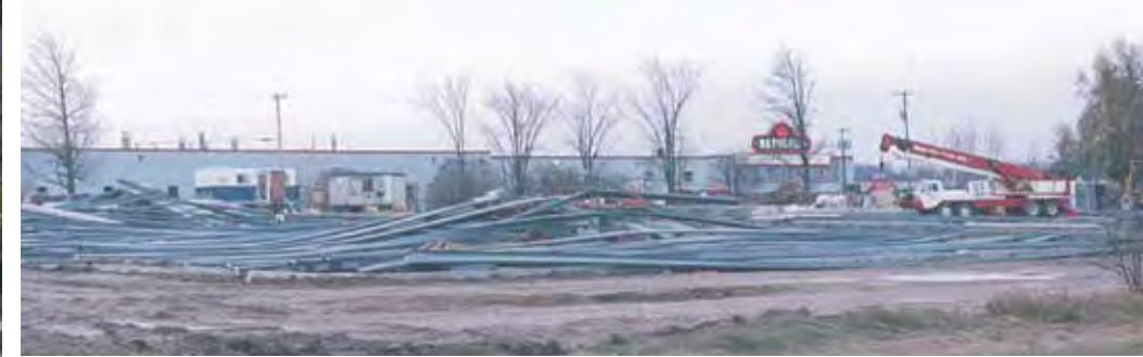
The collapsed steel structure after a windstorm during the construction of the 24 Napoleon Road facility – the contractor had to start all over again.
