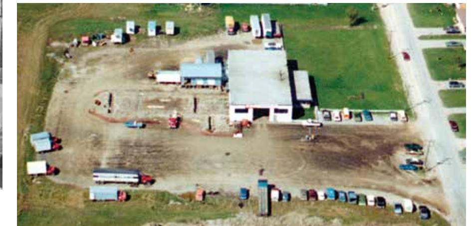
Aerial view of the New Hamburg terminal with the new dock under construction, 1974.
