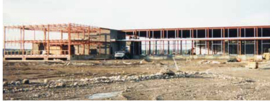
Construction on the new Baden Terminal, 1999.
