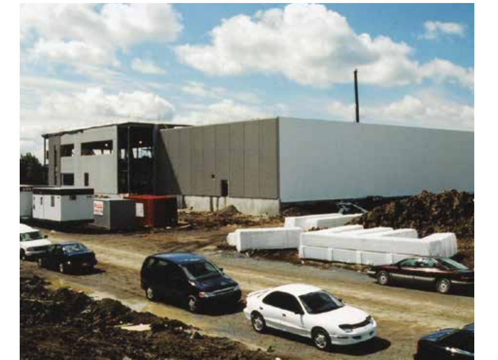
The Erb Terminal in Vaudreuil-Dorion under construction, 2004.
