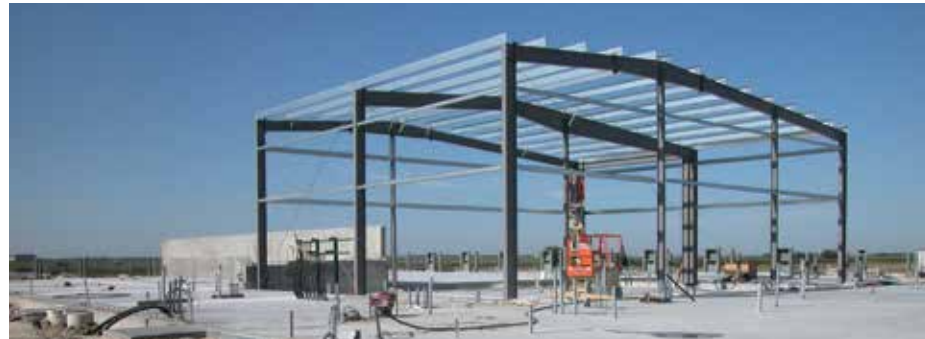
The Winnipeg Terminal under construction, 2009.
