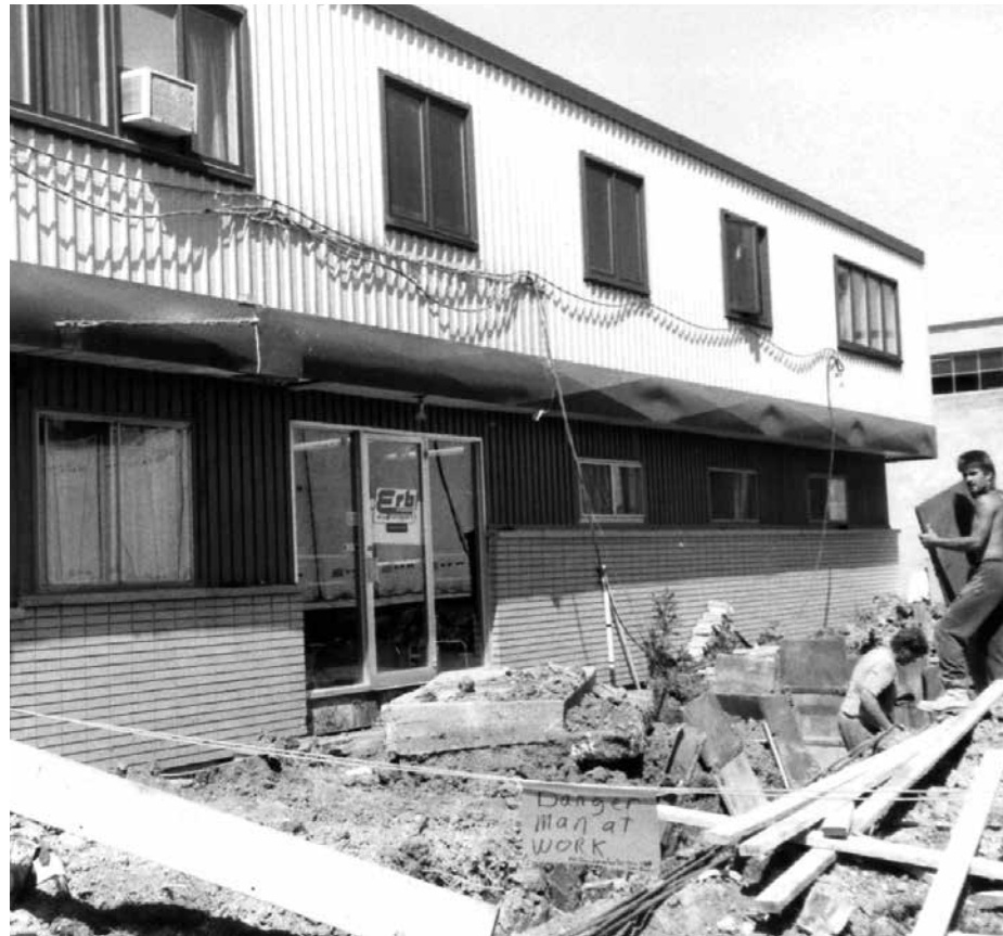
Expansion of the New Hamburg Head Office building.
