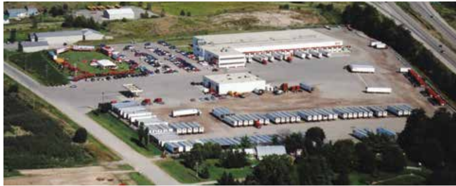
Aerial view of the Baden Terminal.
