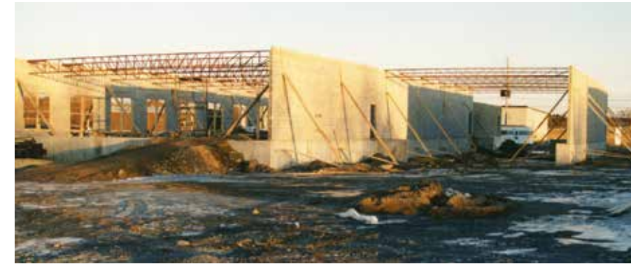
Trenton Terminal under construction, 1990.
