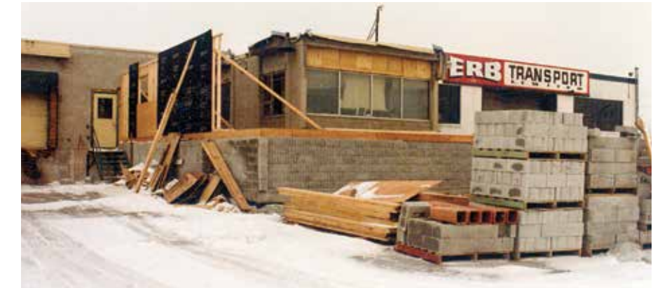
Construction at the New Hamburg Terminal.
