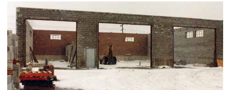
The New Hamburg Trailer Shop under construction.
