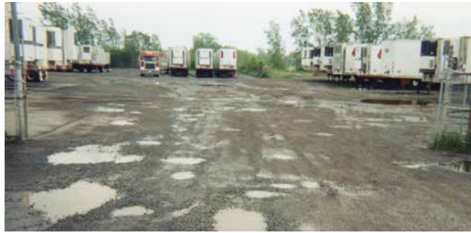
The infamous potholes at the Dorval Terminal.
