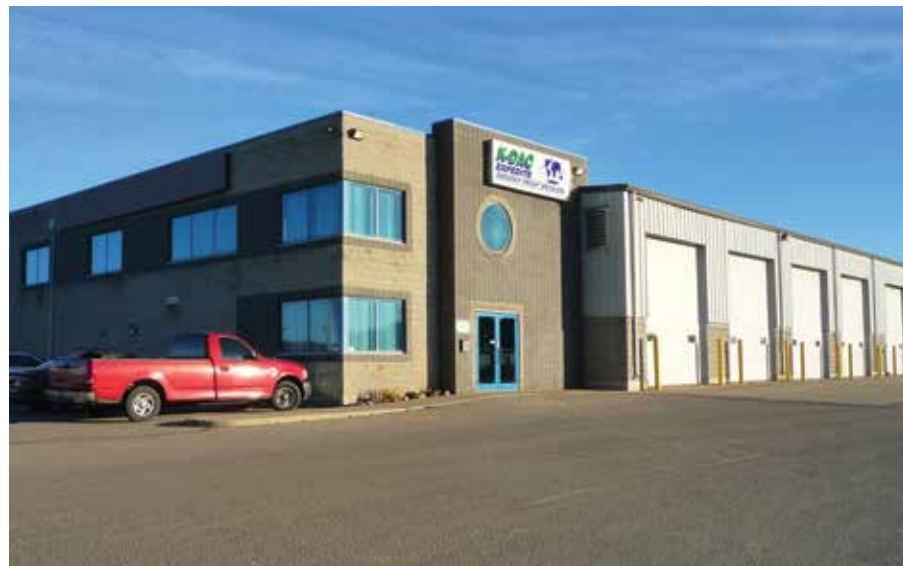
K-DAC's new Sandhills Road head office.
