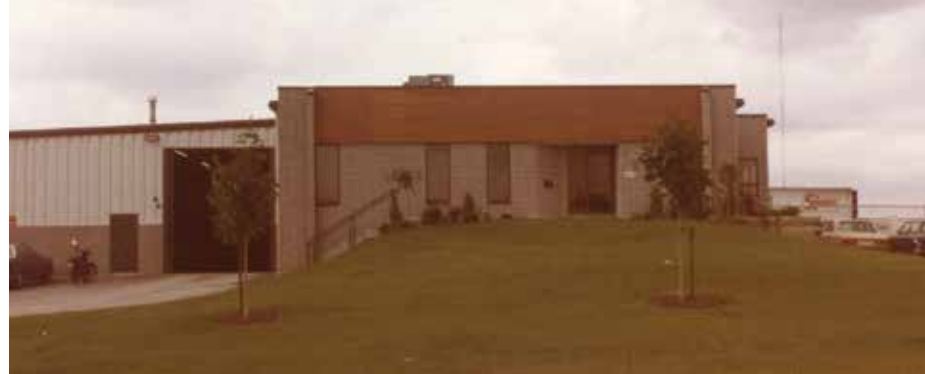
The new Toronto Terminal on General Road completed. Jutzi, Vernon, Richard Roth.
