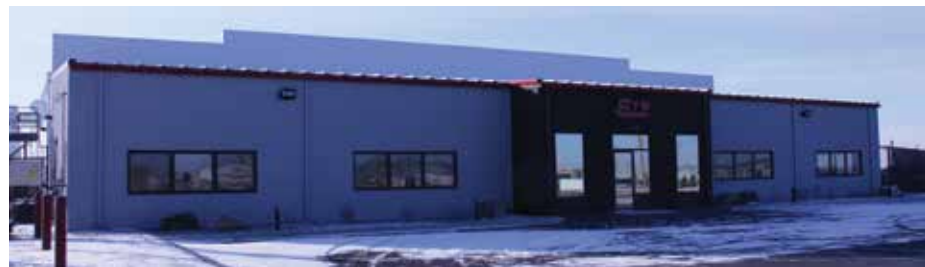
The Winnipeg Terminal completed, 2010.
