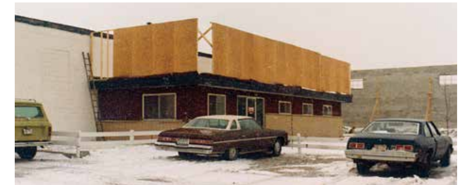
Adding a second floor to the office.
