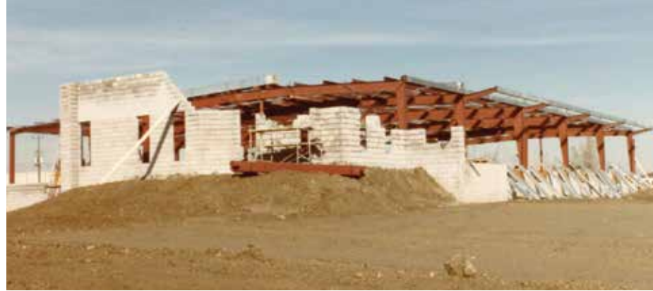
The Toronto Terminal on General Road under construction.
